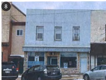
8 140 E Oak St Major Improvements Needed
