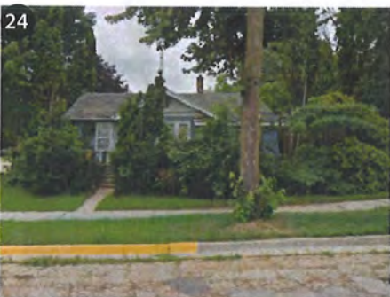
123 W Center St Minor Improvements Needed
