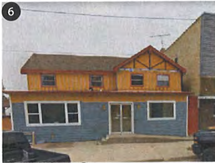
6 130 E Oak St Major Improvements Needed
