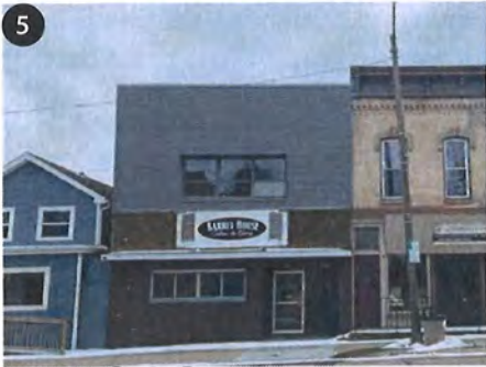
5 124 E Oak St Major Improvements Needed
