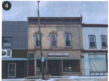
120 E Oak St Major Improvements Needed
