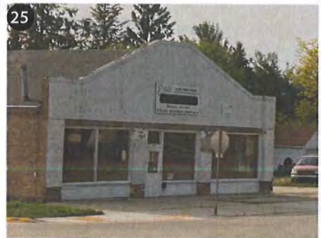
207 West St Major Improvements Needed
