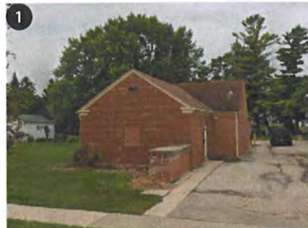
228 E Center St Major Improvements Needed
