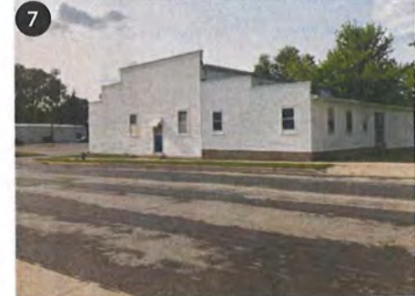
224 N Depot St Major Improvements Needed
