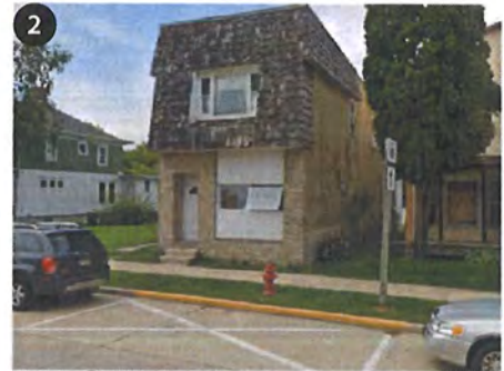
121 S Main St Minor Improvements Needed
