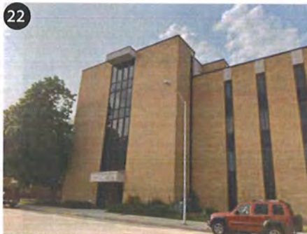
143 E Center St Major Improvements Needed
