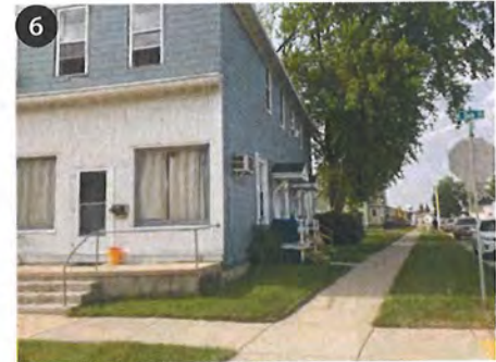
109 N Depot St Minor Improvements Needed
