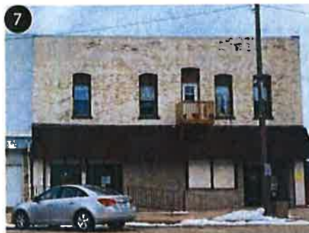
7 140 E Oak St Major Improvements Needed
