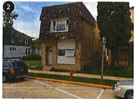
121 S Main St Minor Improvements Needed
