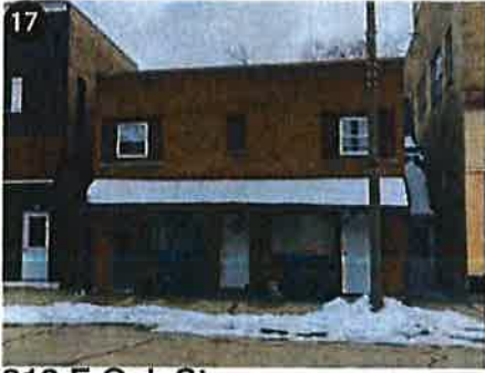
212 E Oak St Minor Improvements Needed
