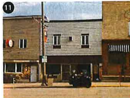
11 156 E Oak St Minor Improvements Needed
