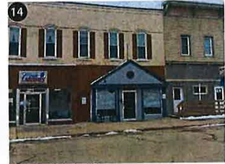
14 166 E Oak St Minor Improvements Needed
