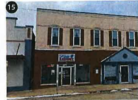
15 168 E Oak St Minor Improvements Needed
