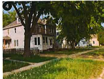
315 E Oak St Minor Improvements Needed
