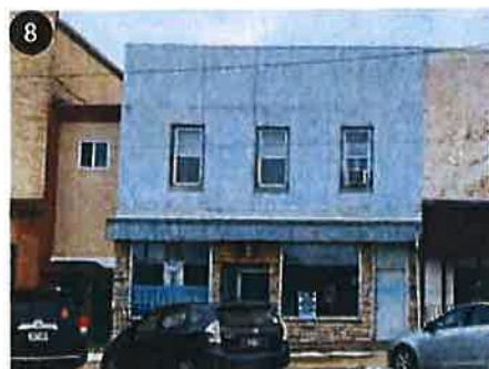
8 140 E Oak St Major Improvements Needed
