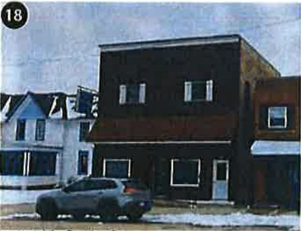
218 E Oak St Minor Improvements Needed
