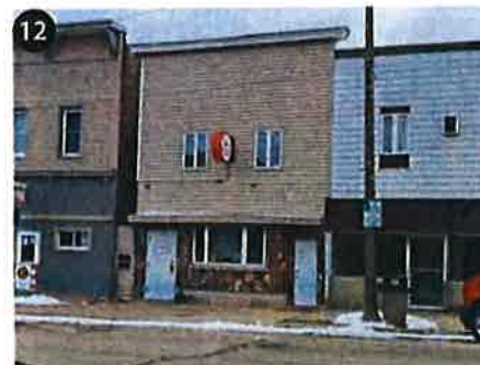
12 160 E Oak St Minor Improvements Needed
