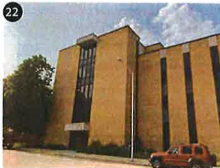
143 E Center St Major Improvements Needed
