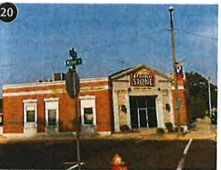
153 E Oak St Minor Improvements Needed
