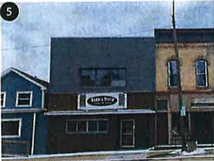
5 124 E Oak St Major Improvements Needed
