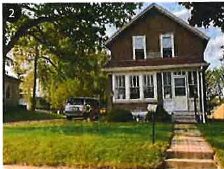
247 E Oak St Minor Improvements Needed
