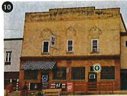
10 150 E Oak St Minor Improvements Needed
