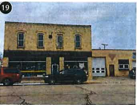
165 E Oak St Minor Improvements Needed
