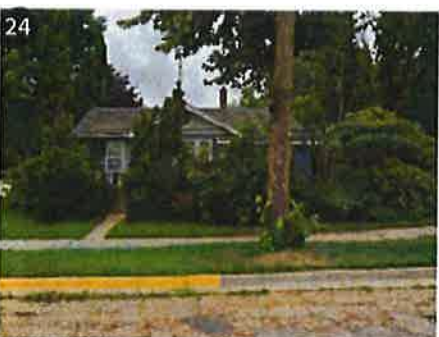
123 W Center St Minor Improvements Needed
