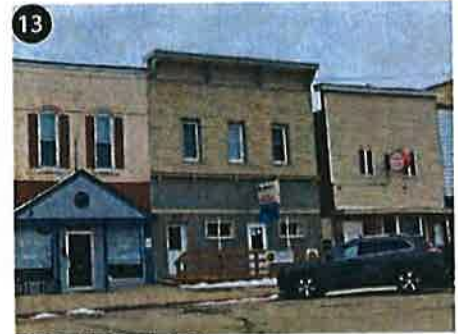
13 164 E Oak St Minor Improvements Needed
