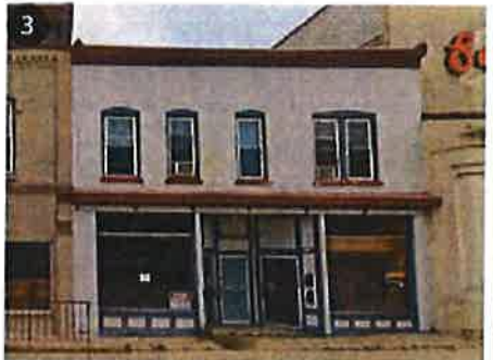
116 E Oak St Minor Improvements Needed
