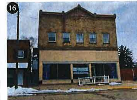
16 208 E Oak St Minor Improvements Needed
