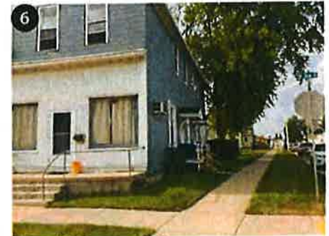
109 N Depot St Minor Improvements Needed
