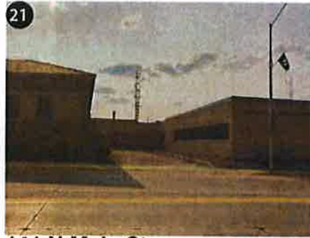
141 N Main St Major Improvements Needed
