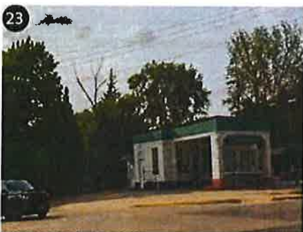
205 N Main St Minor Improvements Needed
