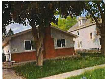
283 E Oak St Minor Improvements Needed
