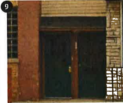
9 148 E Oak St Minor Improvements Needed
