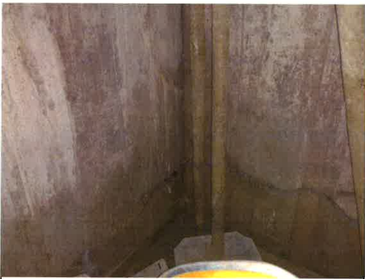
Foundation Southeast corner
