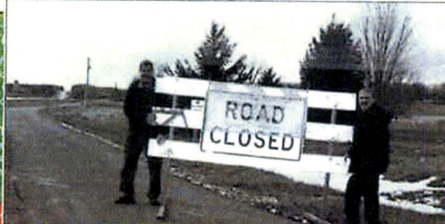
A Gold Star Memorial Trail (GSMT) construction barricade was removed last week by GSMT Project Manager Bill Ehlenbeck, Dodge County Land Resources and Parks Director, on right, and MSA Team Leader and Professional Engineer Mike Laue. (Karen Rouse | DCP)
