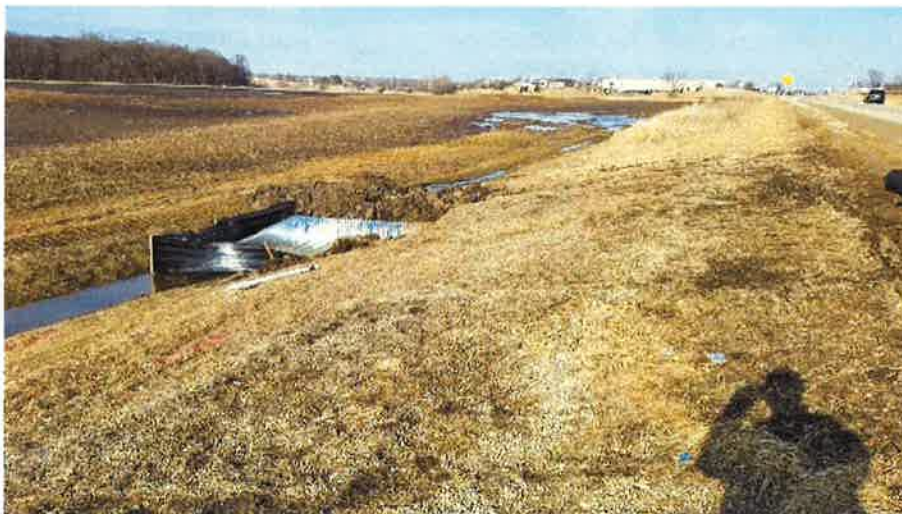
Lengthening existing roadway culverts along STH 28 to accommodate the new trail.
