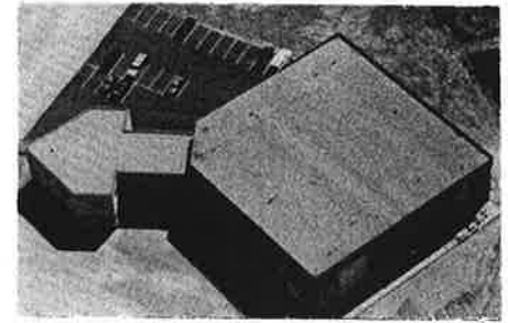
AIRPORT TERMINAL BUILDING
